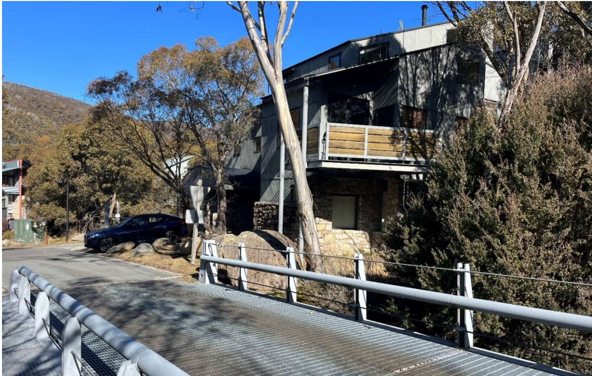
Figure 19: Pinnibar, Crackenback Ridge subdivision
